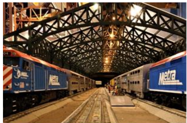
Metra boarding at Downtown Station
