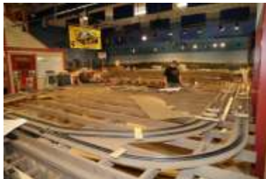
John Billone wires track
