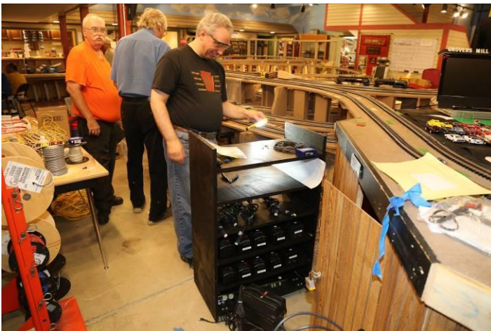
John finishes power and Legacy/TMCC controls
